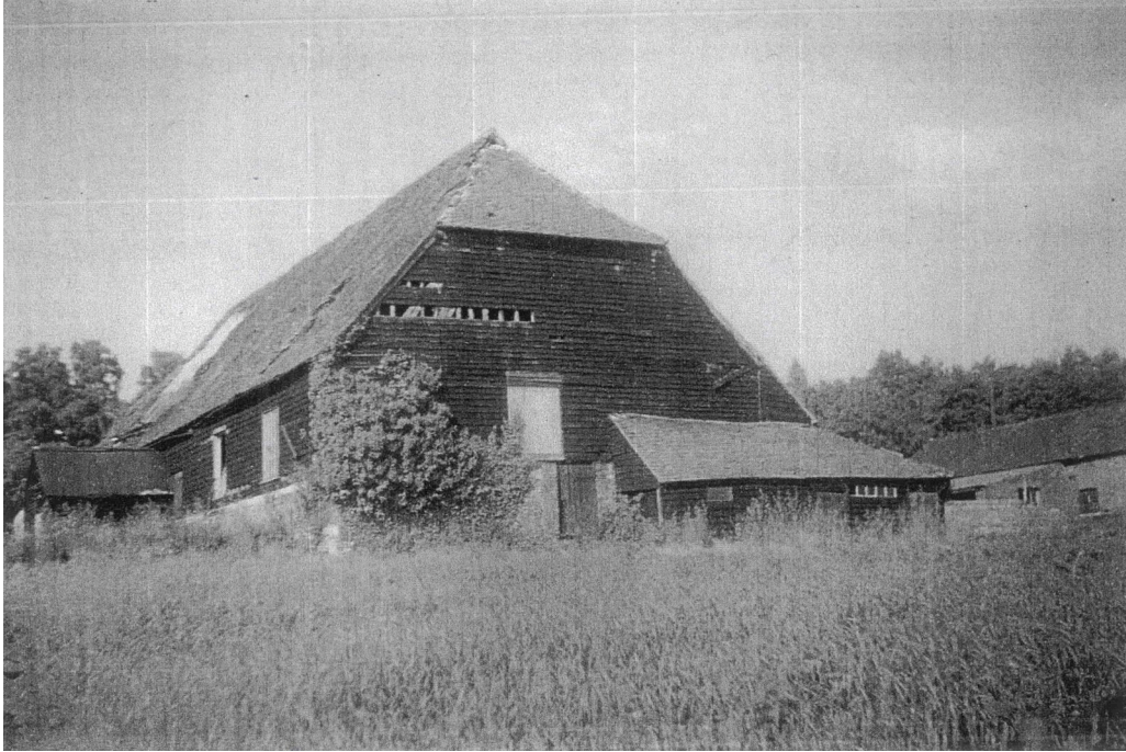
Fig. 13 Croxley Great Barn, South Elevation Showing Demolished Upstand Structure circa 1972 Photograph courtesy of Three Rivers Museum Trust.
