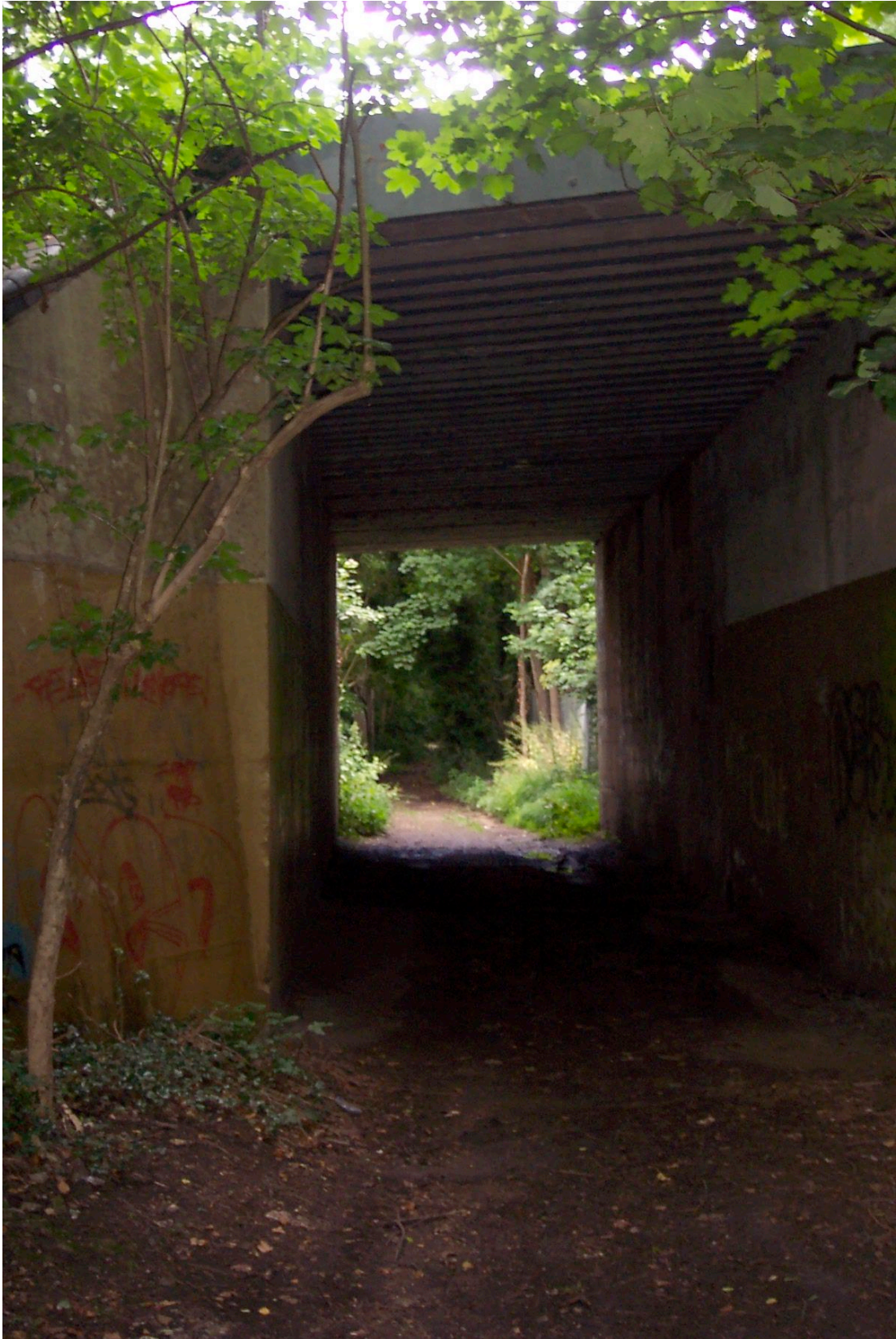
Fig. 39 Croxley Great Barn, Access Tunnel from Lavrock Lane to Playing Field
